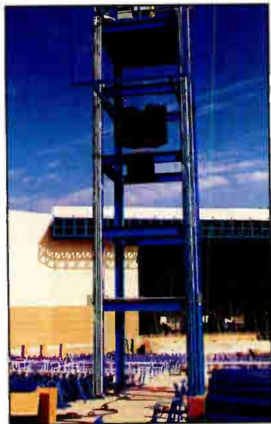
The Pavilion's stage is 100 feet wide, 68 feet deep and 48 feet high. The flying grid is rated at 105 tons, and most acts will choose to fly their P.A., says production manager Nick Kotos. However, there are two 40x15-foot stage wings that can be used for stacked sound, or as staging areas. Loading docks are said to accommodate five 18-wheelers simultaneously.
