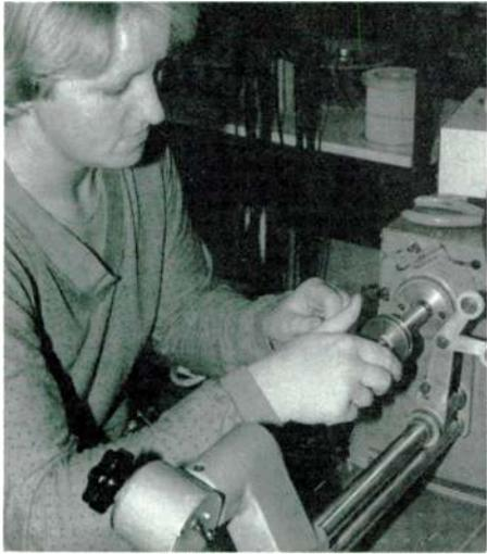
Fig. 9. Lilian Smith assembles a mandrel preparing to wind one of the 14 delay inductors in the Quad-63 speaker.
