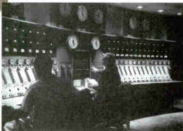
Twenty-six programs can be fed through the master control console simultaneously at Voice of America.
