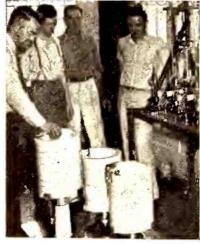
ENGINEERS—Of WMBD, Peoria, Ill., examine tube-coolers in front rectifier rack while installing new 5,000-watt Western Electric transmitter, expected to go into operation Sept. 15. Left to right are Chief Engineer Ted Giles and Engineers Bob Connor, Bert Giles and Harry McCormick.
