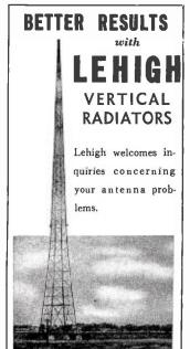
Illustrated: 242 ft. insulated Lehigh Vertical Radiator at WKAQ. San Juan, P. R., built to withstand 200 mile indicated wind velocity.
