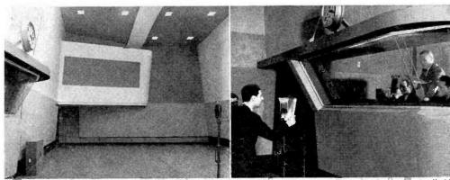
SLANTING WALLS—Are used in the studios of the new CBS building in Hollywood, dedicated April 30. All eight studios have this feature, designed to eliminate acoustical flutter. Even the projecting control room windows are slanted to avoid reflection. While as many as five colors are used in each studio, one color predominates in each case. Double walls isolate the rooms from the rest of the building.
