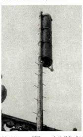
**READY**... **AIM**... but this skyrocket styled FM antenna installed at WGHF New York doesn't fire, it just radiates. And according to Capt. W. G. H. Finch, president of Finch Telecommunications and personal owner of the FM station, it effects a concentrated radiation toward the horizon, with less power going skyward and into immediately adjacent area where not needed [BROADCASTING, Nov. 19].
