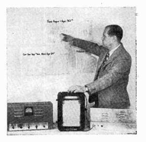
LAUGH-GRAPH is one purpose of the newly-developed electronic instrument for measuring audience sound reactions, demonstrated recently by Ernest M. Walker, president of Ernie Walker Inc., New York. Device picks up sound through sensitive microphone over audience and by means of electronic impulses pens off time intervals and units of sound volume. Charting service will be offered agencies, sponsors and production services.
