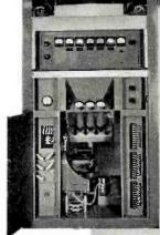
One of the Du Mont television transmitter units - 5 KW Visual Amplifier, with three built-in cathode-ray indicators.
