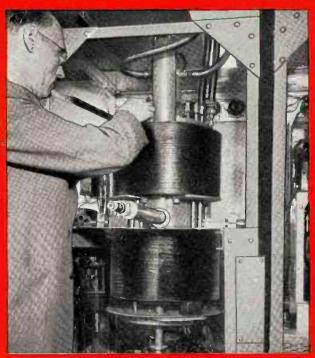
High-Power UHF Klystron Tube. A successful solution to the difficult problem of high power at UHF. Designed and built to G-E specifications, this tube's remarkable amplification and extreme stability actually make high-power UHF television a reality.
