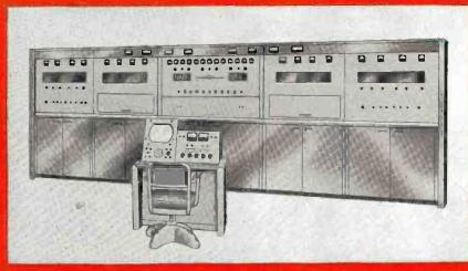
World's Most Powerful UHF Television Transmitter. This 12 kw unit offers a unique trequency control system. One crystol oscillator controls both the visual and the aural carriers, locking them together with a fixed separation of 4.5 mc. A number of broadcasters have already placed orders for this UHF transmitter.
