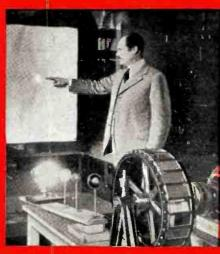
First Television 'STransmitter' is demonstrated by its inventor. Each of the 24 mirrors mounted on a wheel of the machine was set at a different ongle to felevise an image before 7 photocells.
