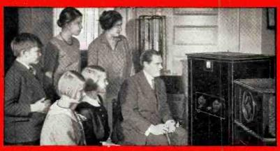
First Home TV Receiver. In 1927, at Schenectady, Dr. Alexande son reveals his console model with a tiny 3" screen. The receiver used a rotating perforated disc to scan the image. Sound was received on a different wave length through speaker at right.
