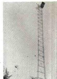
THIS is new two-tower array of the Bell microwave relay system completed for WJIM-TV Lansing, Mich., and part of the \$250,000 Bell system completed by AT&T. Signal is beamed from Detroit to 274-ft. tower at Milford, to a second tower at Danville, to receiver in Lansing and then to the WJIM-TV tower.
