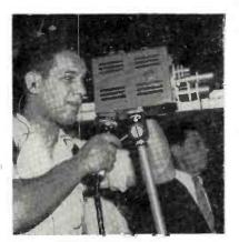
WALKIE-LOOKIE, new video camera developed by RCA, was used on the convention floor by NBC at the opening session Monday when the New Jersey delegation was polled on the crucial rules question. The device, which was being tested as the roll call took place, was moved quickly into action for a three-minute network feed. It was premiered for the press July 5.
