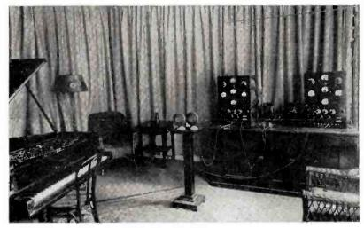
WDRC, operating as binaural station in 1924, shows studio containing right-ear and left-ear microphones and transmitters.
