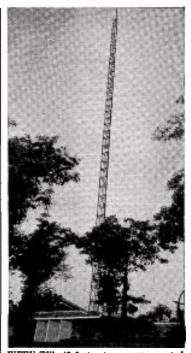
WEEU-TV's 43-foot antenna was mounted on a 365-foot guyed tower atop Mt. Penn, directly overlooking Reading from the east.
