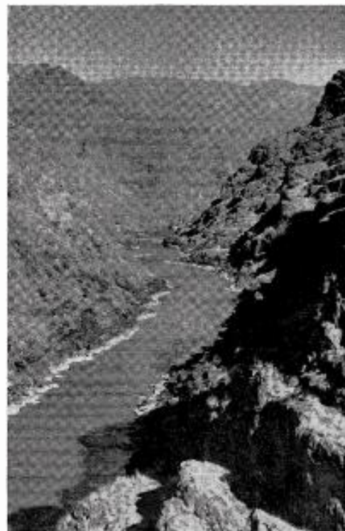
SOME DAY SOON, Northwesterners hope, this Pleasant Valley site on the Middle Snake River will feed its swift waters through hydroelectric generators.
