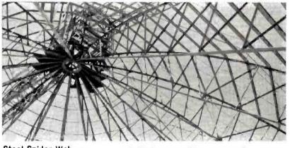
Steel Spider Web. If you ever needed it, here's proof that amazing things can be done with steel. This is an 83-foot-high dome for a potash storage building that will be covered with steel sheets. This complicated structure was *prefabricated* and erected by American Bridge Division of U. S. Steel.
