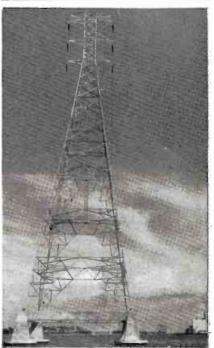
High Line At Low Cost. These gigantic electrical transmission towers are 198 feet high—because they must provide 100 feet of clearance for ships passing underneath in Old Tampa Bay, Florida. By using a special USS MAN-TEN High Strength Steel, 6½ tons were trimmed off the weight of each tower. The total money saving for four towers amounted to \$7,200... far more than the slight extra cost of the high strength steel. Another job well done with steel!
