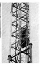
(right) Rated for a load of 750 pounds, will comfortably accommodate two people. Car stops automatically if door is opened, will not start until it is closed. Supported by a double set of cables, either one of which will hold the car and its full load.
