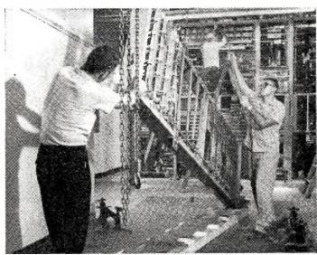
STEADY AS SHE GOES. After uncrating, the intricate frames of switching equipment are hoisted upright and placed in position. One hundred ninety such frames are being installed in Vincennes, bringing dial service to over 7,000 telephone customers.
