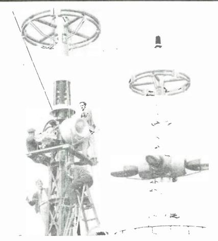
NEW TELEVISION antenna being built for operation by RCA-NBC atop the Empire State Bldg., New York, Left photo shows antenna being erected for test at the RCA Communications laboratories at Rocky Point, Long Island, Right photo shows how it will appear when installed.
