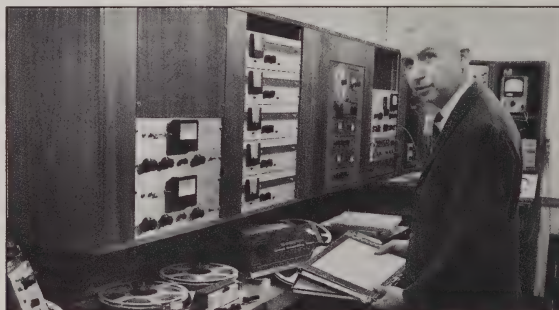
Jack Mullin returned from post-war Germany with two Magnetophon audio recorders and several reels of paper-backed audio recording tape. Mullin worked with Bing Crosby to pre-record Crosby's nationwide radio variety show—this time with audio tape by 3M, with whose recording tape division he later joined.
