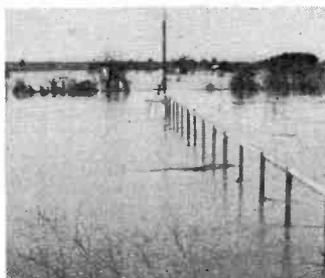
**SURROUNDED** by flood waters of the Tombigbee River for the second time within a year, the antenna tower and runway for the transmission line of WCB1 Columbus, Miss. are visible. Base of WCB1 tower is on a concrete foundation 15 feet above ground. WCB1 engineers used boats to read antenna meters, visible above the water.
