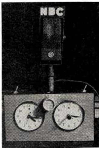
CONTROL ROOM CLOCKS like this pair, operated by the toggle switches seen above them, are standard WTAM equipment for timing rehearsals. The one at left is used for total timing, may be stopped when rehearsals must be interrupted. One at right, used as stopwatch, times interruption.
