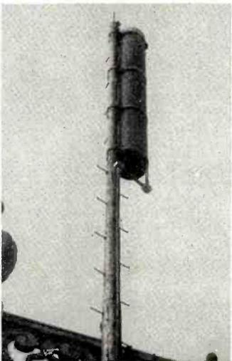
**READY . . . AIM . . .** but this skyrocket styled FM antenna installed at WGHF New York doesn't fire, it just radiates. And according to Capt. W. G. H. Finch, president of Finch Telecommunications and personal owner of the FM station, it effects a concentrated radiation toward the horizon, with less power going skyward and into immediately adjacent area where not needed [BROADCASTING, Nov. 19].
