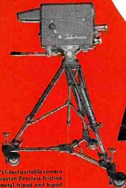
Television's finest portable camera mount. Houston-Fearless friction head, all-metal tripod and tripod dolly. For studio or field use.
