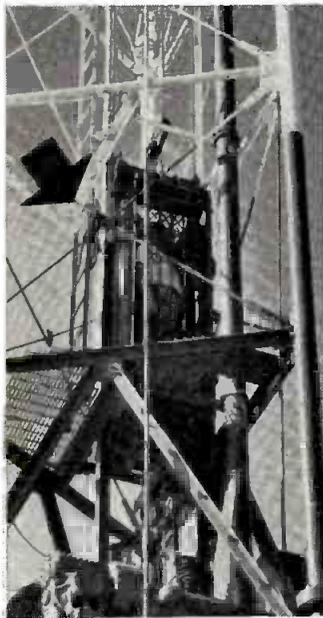
Tower and antenna inspection and maintenance are no problem. A special-design two-man Marshall service elevator installed within the tower permits easy access to any level. This completely enclosed, automatic elevator features ground-to-cab telephone communications and can be controlled from either the cab or lower landing.
