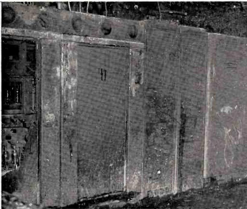
Blackened ruins of the WKRS transmitter room. Lightning started the fire in the switch panel at left.
