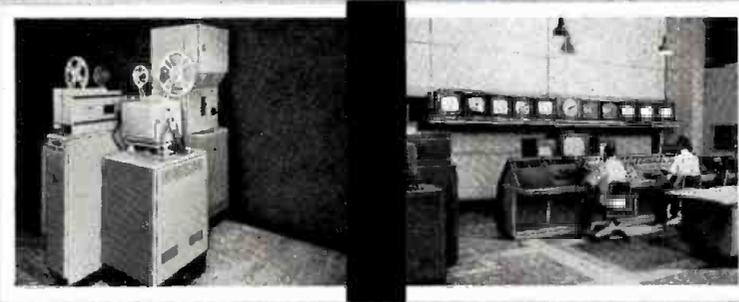
• The Multi-Scanner installation in control room of WITI-TV provides complete color and monochrome pickup facilities for film and slides. In addition, the Multi-Scanner light source is used as a fixed camera for the adjoining Studio No. 2.
