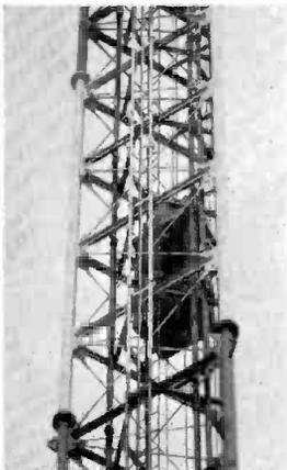
(right) Car is fitted with spring-loaded nylon rollers which engage the guide rails, prevent car sway and insure smooth operation.
