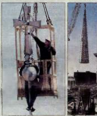
At left, Jimmy Hoek, standing, and Mary DeJure, kneeling, accomplish the tough job of threading an 8-foot-tall, steel-as-steeled casket into a mast atop the new Old Stone Church steeple in Public Square. An aluminum replica of the original spire, right, is shown in place atop a steel tower anchored to the church. The mast made two turns to 200 feet before being lowered to maneuver the 300-pound casket into place and 22 mph winds. For a detailed look see tomorrow's religion section.
