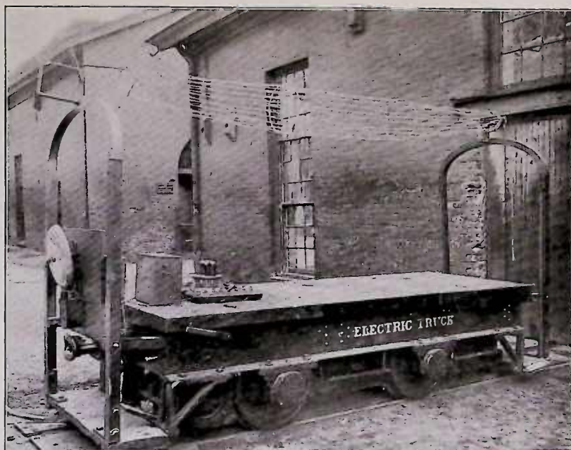
Wireless Controlled Electric Truck, designed and operated by Dr. Frederick H. Millener, E.E.
