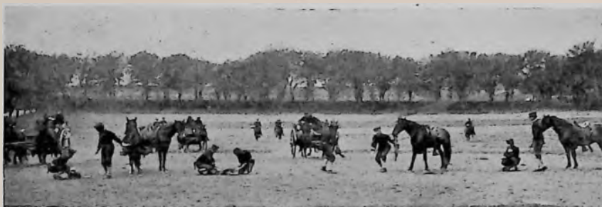
REELING UP WIRE WITH AUTOMATIC CARTS
