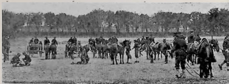
LAYING FIELD WIRE
