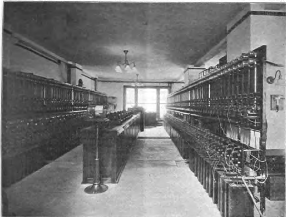
Figure 2.—TAPE TICKER AND PAGE PRINTER SWITCHBOARDS. STOCK QUOTATION TELEGRAPH COMPANY, NEW YORK.
