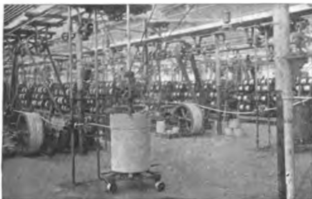
Figure 2.—STRANDING MACHINES AND CABLES IN PROCESS OF BEING FORMED INTO CORE.
