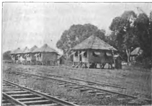
Section Houses, Philippine Railway.
