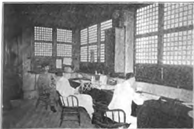
Sub-station Philippine Railway, Iloilo.
