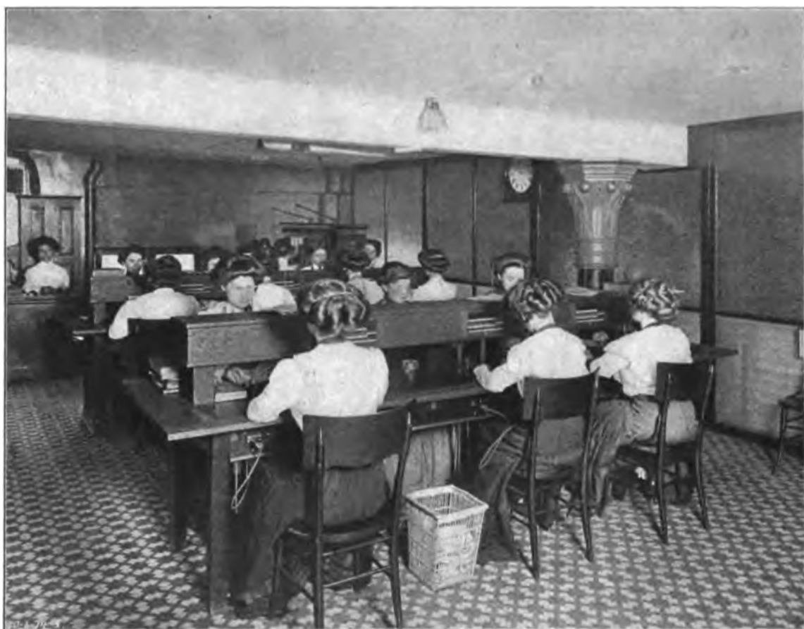
VIEW OF TELEPHONE GALLERY IN CHICAGO OFFICE OF WESTERN UNION TELEGRAPH COMPANY.
