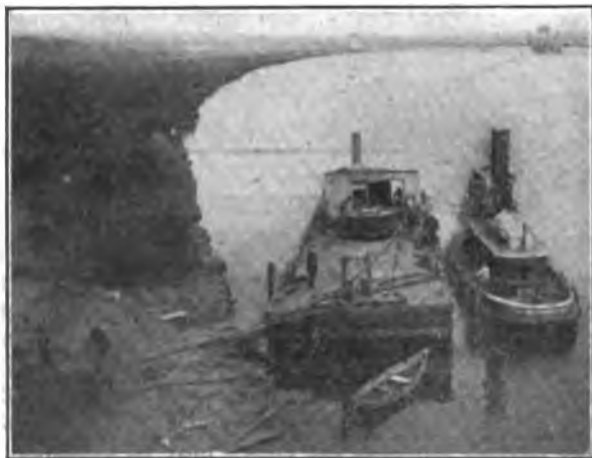
UNREELING SUBMARINE CABLES FROM BARGE.
