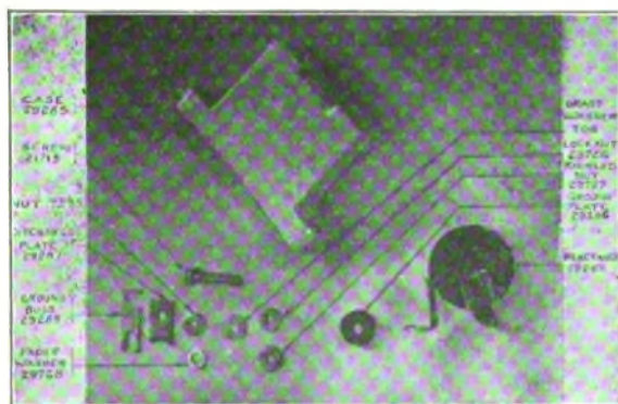
DETAILS OF ARRESTER.
