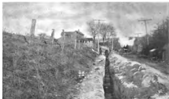
FIG. 2.—TRENCH READY TO RECEIVE DUCTS.
