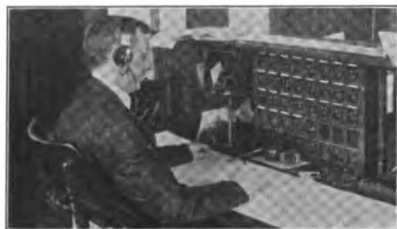
FIG. 1.—TRAIN DISPATCHER'S OFFICE EQUIPMENT AT ROCHESTER, N. Y.
