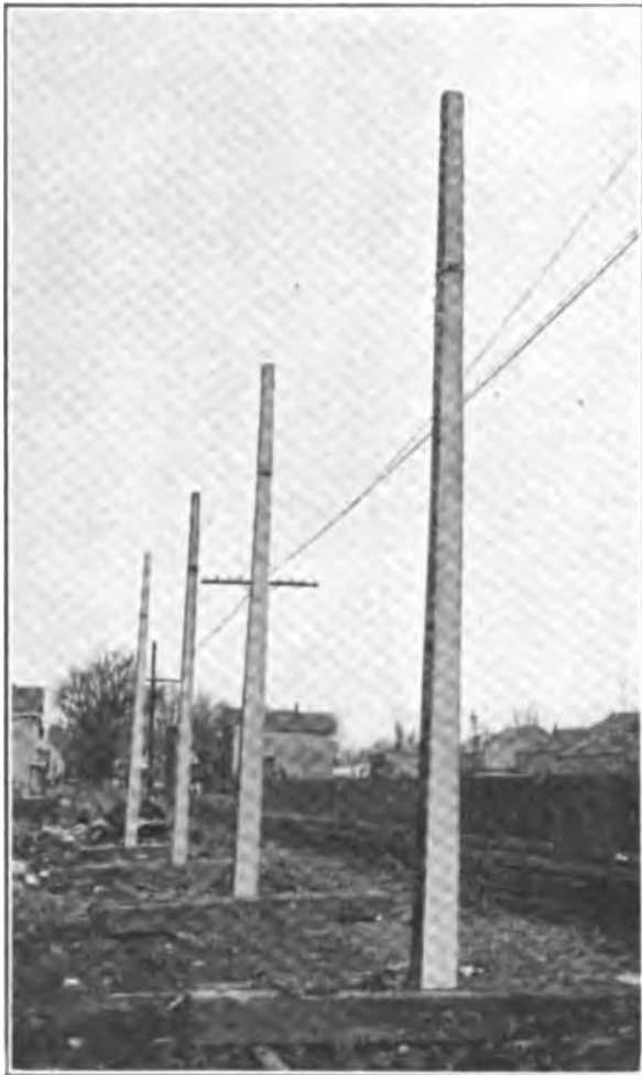
FIG. 1.—ROW OF THIRTY-FOOT POLES ERECTED IN BOGGY GROUND.
