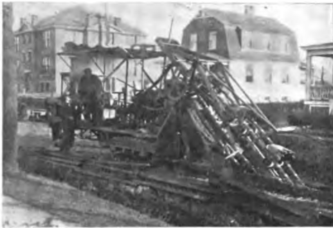
FIG. 1.—TRENCHING MACHINE AT WORK.
