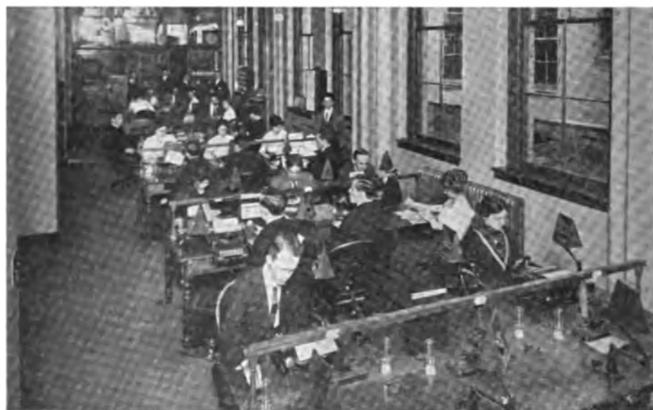
FIG. 2—VIEW OF TELEGRAPH OPERATING ROOM, NEWARK, N. J.
