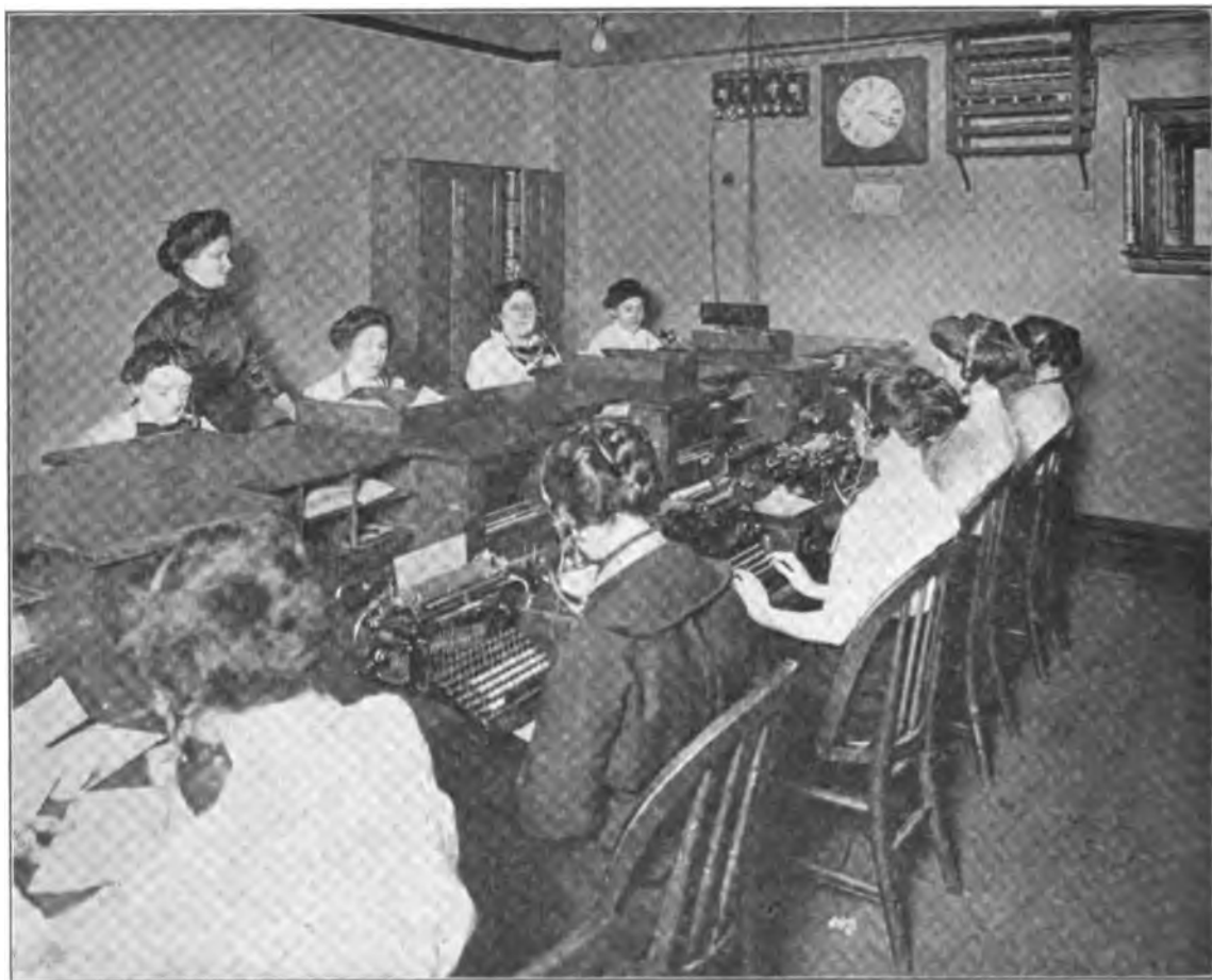
TELEPHONE RECORDING TABLES AT PHILADELPHIA WESTERN UNION OFFICE.
