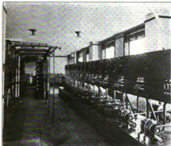
FIG. 5—MOTOR-GENERATORS AND CABLING IN REAR OF TEST BOARDS
