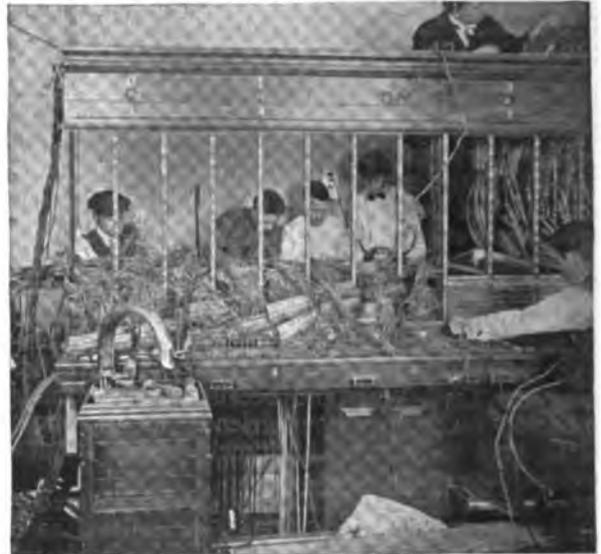
FIG. 2—WIREMEN REPLACING BURNED AND WATER-SOAKED CABLING TERMINATING IN THE PARK SWITCHBOARD, WORCESTER, MASS.
