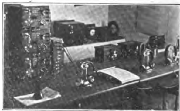
RECEIVING STATION AT EUREKA, S. D.
