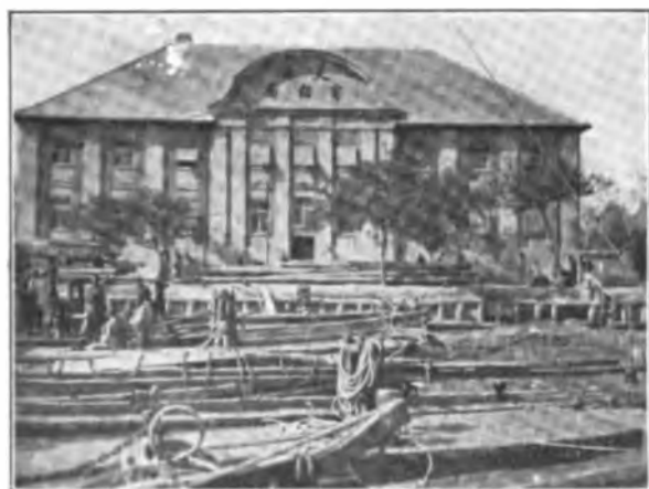
FIG. 1—TELEPHONE CENTRAL OFFICE BUILDING, TIENTSIN.
