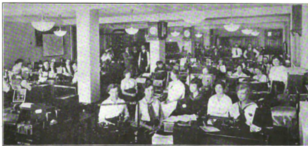
MAIN OPERATING ROOM, HELENA, MONT.
