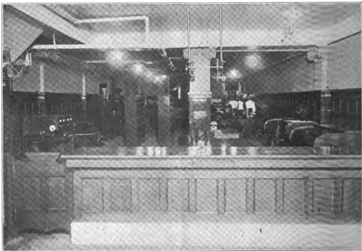
JACKSONVILLE, FLA., OFFICE, POSTAL TELEGRAPH-CABLE COMPANY.
