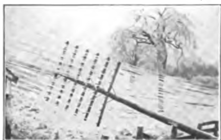
FALLEN POLE WITH SLEET COVERED WIRES.
