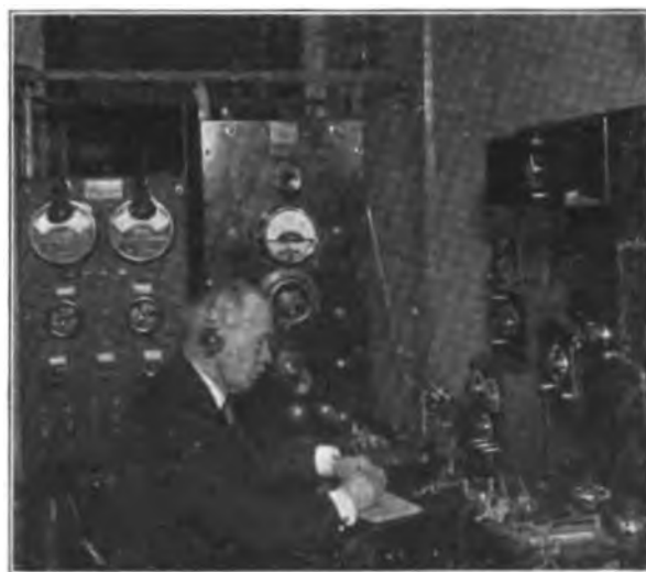
FIG. 1.—LACKAWANNA WIRELESS OPERATING ROOM.
