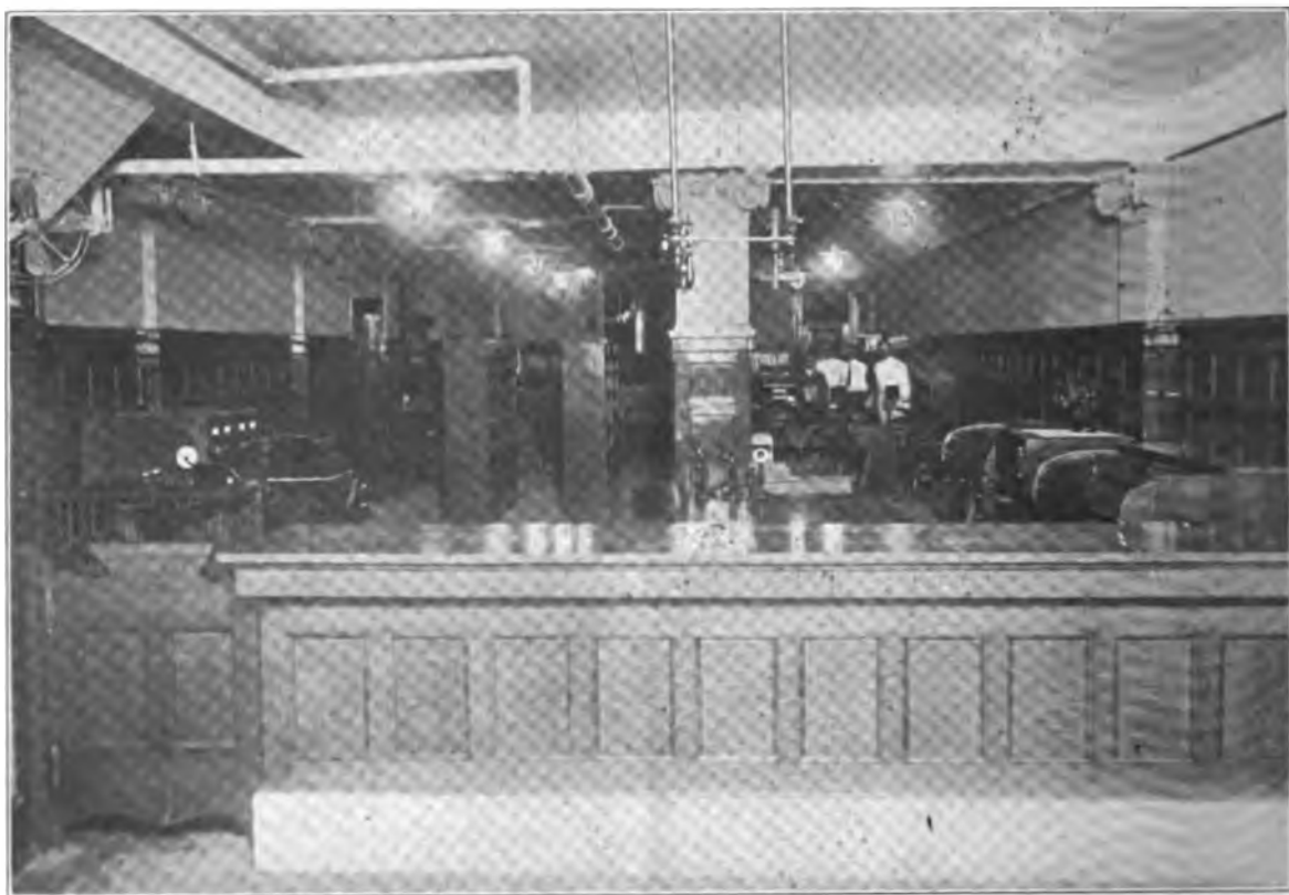
JACKSONVILLE, FLA., OFFICE, POSTAL TELEGRAPH-CABLE COMPANY.
