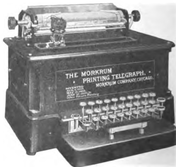
FIG. 2—KEYBOARD AND HOME RECORDER.
