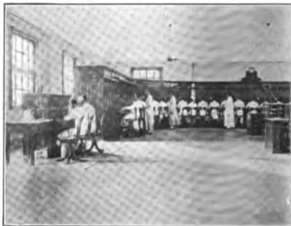
FIG. 2—INTERIOR TIENTSIN CENTRAL OFFICE.
