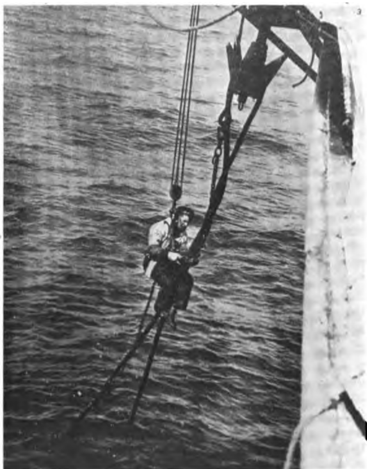
PLACING "STOPPERS" ON A PICKED-UP CABLE TO PREVENT IT SLIPPING BACK INTO THE SEA.
