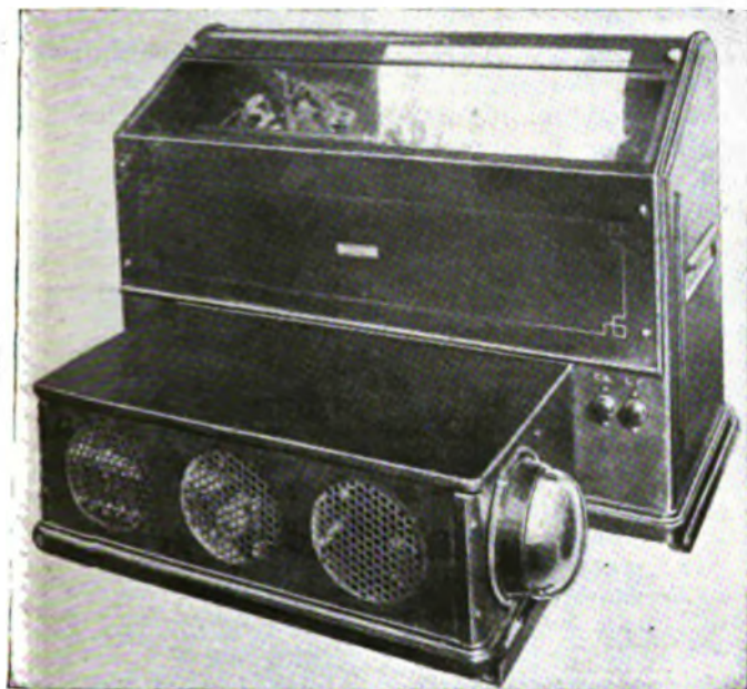
FIG. 4—RECEIVING PRINTER.
