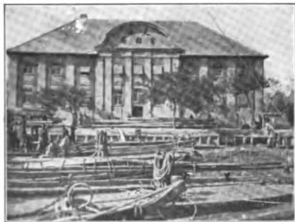
FIG. 1—TELEPHONE CENTRAL OFFICE BUILDING, TIENTSIN.
