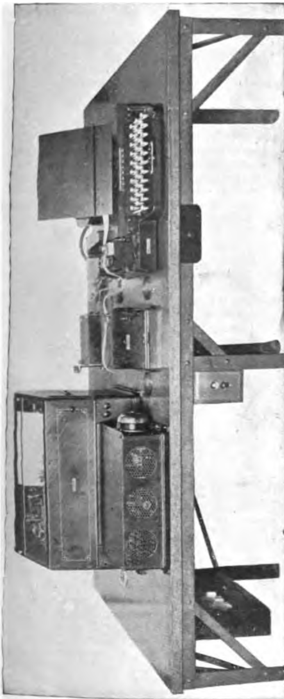
FIG. 14.—COMPLETE MULTIPLEX TABLE EQUIPMENT.
