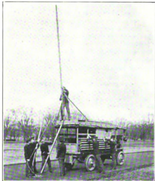
FIG. 2—ERECTING A MAST ON A TRACTOR.
