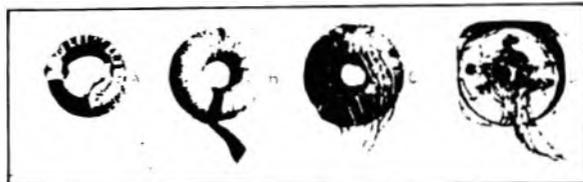
FIG. 1—STAGES IN THE MANUFACTURE OF A REPEATING COIL. A, Iron Core Wrapped with Tape; B, Primary and Secondary Windings in Place; C, Coil Taped and Waterproofed; D, Coil in Position, Impregnated with rosin.
