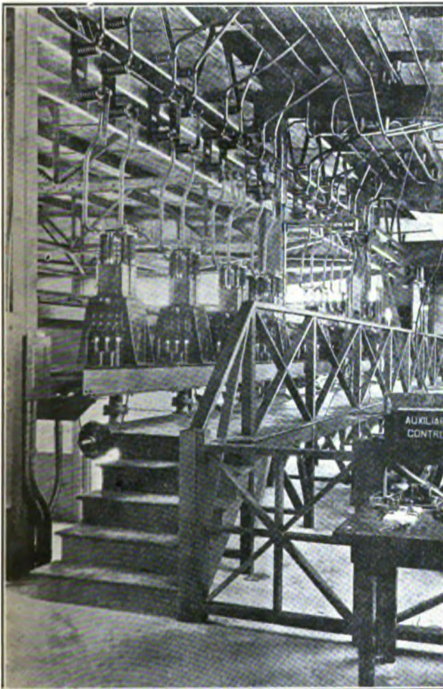
FIG. 5—HIGH-SPEED AUTOMATIC SENDING KEYS AND BUSES IN TRANSMITTING STATION.
