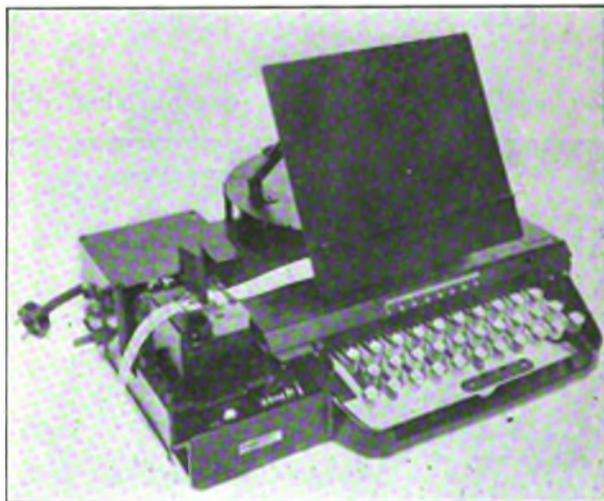
FIG. 1—KEYBOARD PERFORATOR.
