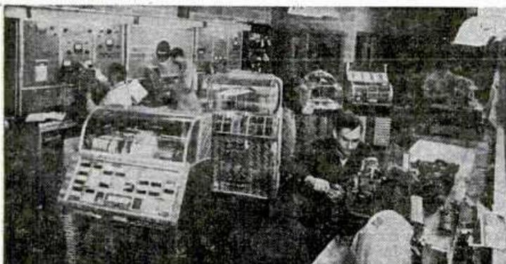
PHONOGRAPH SELECTED for export at Atlas Music Company, Chicago, undergoes complete overhauling. Here, in the firm's modern service department, trained mechanics and technicians check record mechanisms and all electrical connections with special testing apparatus. Panel at the rear of the shop tests everything from ohm and volt output to tubes and sound frequencies.
