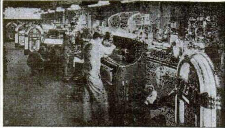
**PHONOGRAPHS PREPARED FOR EXPORT.** The first step for a Davis Distributing Company phonograph marked for export is in the firm's modern service department. Here machines are set up as on an assembly line, checked inside and out for needed adjustments and given a complete overhauling.
