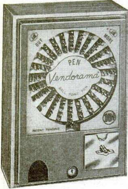
Victor's revolutionary and unique method of selling ball point pens. The revolving action displays all pens and assures positive delivery. Capacity 168 ball point pens, vending at 10c each.
