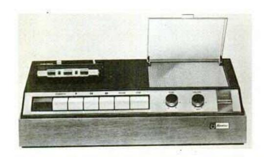
First home development of the Philips cassette equipment was this table model seen here bearing the Norelco logo. Fold-down audio reflector maintains minimum dimensions of the concept.
