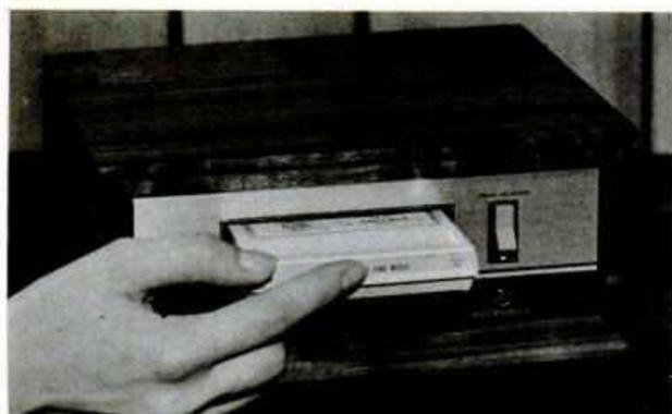
MOTOROLA unveils its 8-track cartridge plug-in attachment, model CP7C, at the Consumer Electronics Show.
