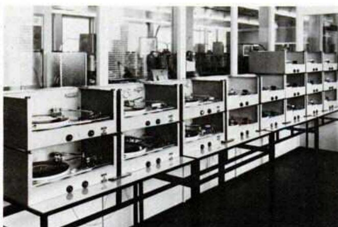
A battery of specially adapted record players in the quality control department of the No. 1 Deutsche Grammophon factory in Hannover. The players are equipped with a second arm which records defects on a slip of paper.
