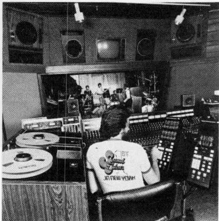
**NEW DIGITAL**—Jim McCurdy, chief engineer for New York's Sound Ideas Studios, mans new 3M 32-track digital recording equipment as r&b group BT Express give it a workout. The Manhattan facility becomes the first New York studio to receive a 3M digital mastering system, consisting of four-track and 32-track recorders.
