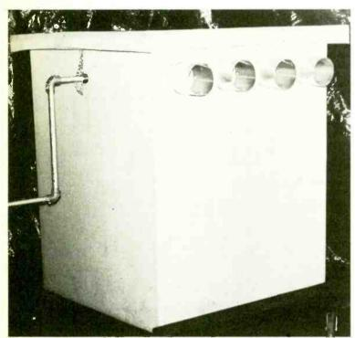
STAR FOG-Starfire Industries of Schenectady, N.Y. has developed a 140 gallon, heat resistant dry ice fog machine for use in special effects for discos and other theatrical environments. The unit features two, 3,000 watt heaters. has a 525 CFM blower, and holds up to 160 pounds of dry ice. Casters for easy mobility of the unit are optional. Suggested price is \$829. Thirty and 70 gallon versions are available at \$329 and \$529 respectively
