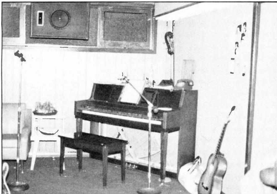
This photograph shows how the windows have been covered with cork to prevent light from entering. The walls on both sides of the room have been covered with cork but one wall was wood panelling for the purpose of reflection. This gives a live sound to the room.
