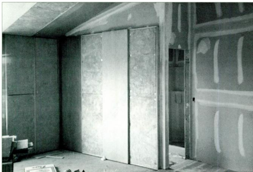
FIG. 3: The bass traps are built using wooden frames and plywood panels, sealed with caulk to make them airtight. The gap below each frame allows room for the carpet, which is not yet installed.
