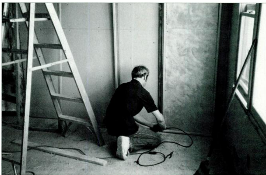
FIG. 4: Master carpenter Rick Castillo attaches a bass trap to the wall with toggle bolts.
