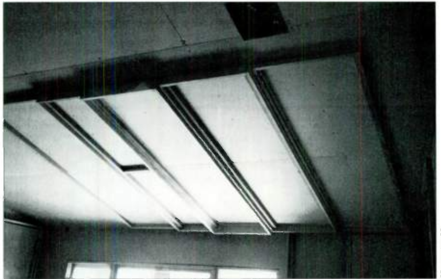
FIG. 2: The bass-trap frames are assembled and mounted before attaching the fiberglass and plywood panels. These traps are on the ceiling over the mixing desk.
