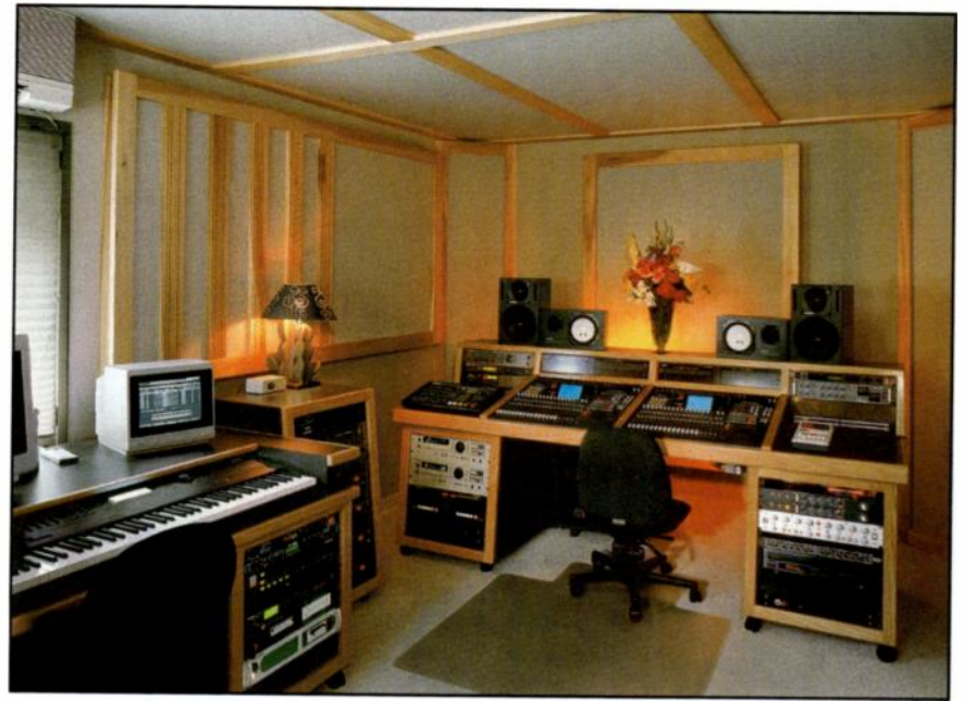
Christopher Cross's personal studio. Notice how sound absorbers are strategically placed on the walls and ceiling as well as in the corners.
