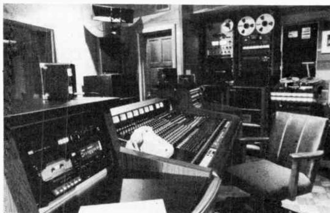
We now master on the Ampex ATR-102, the choice of most major studios. With the Eventide 949, Harmonizer, 2 Lexicon Prime Time Digital Delays, EMT Stereo Plate Tube Reverb, and U47 Tube Microphone, we make your vocal tracks outstanding. We now have a Fender Rhodes 88 in addition to our Yamaha C3 Piano, Hohner D6 Clavinet, and Arp Omni Synth and string ensemble. We are noted for our great studio drum sound!
