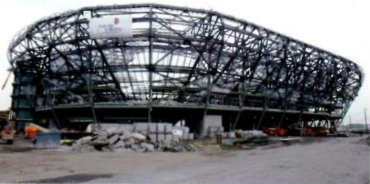
**THE STEEL SUPERSTRUCTURE** of the New York Red Bulls soccer stadium is under way in Harrison, N.J. Construction workers have placed the last piece of structural steel on the soccer-specific stadium, which is set to open in 2010.
