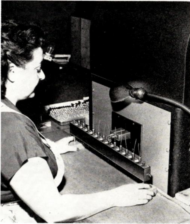
High frequency soldering of glass-to-metal ends hermetically seals subminiature "Glas-seal" types.
